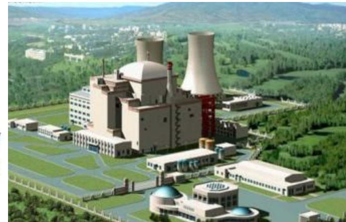
Figure. In a nuclear power plant, fission energy creates heat, which is used to produce steam. The steam drives a turbine, which generates electricity.
