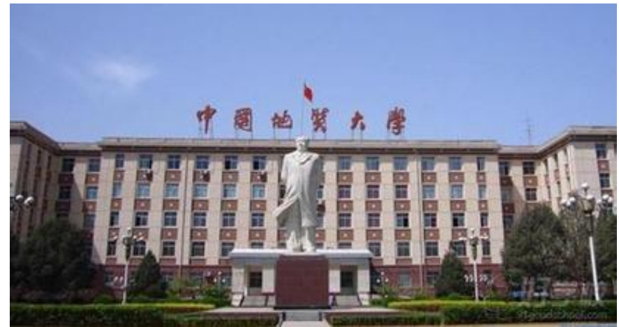
Library Building, China University of Geosciences
